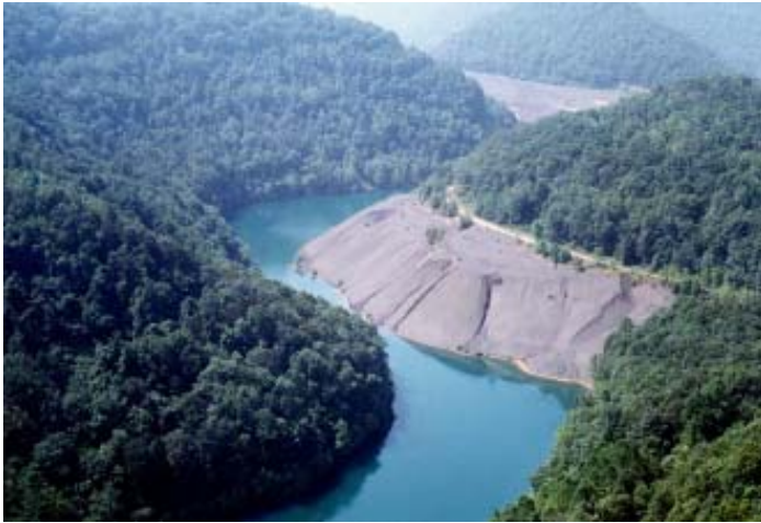
Before reclamation - This aerial view looking west clearly shows the pile's steep slopes with eroding refuse leading down to the dangerous impoundment.
